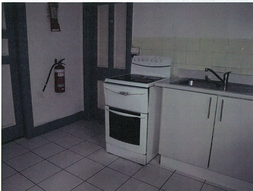
PHOTO 16: PRESENT KITCHEN WITH RETAINED DOORS AND ARCHITRAVES Cream tile possibly later c 1960's. Joinery, stove etc late 20 th Century
