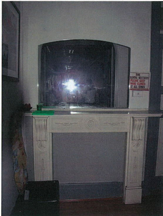
PHOTO 12: GROUND FLOOR - ALTERED SOUTH ROOM – Original fireplace closed off
