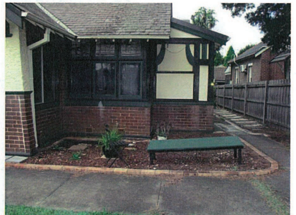
Photo 5: South western corner facing Lucas Road.
