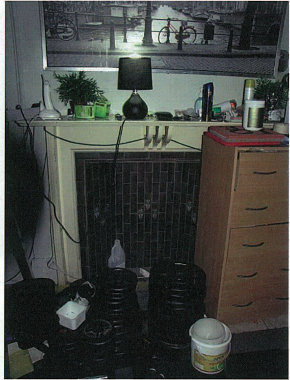
PHOTO 11: ORIGINAL TILED FIREPLACE RECESS – Possibly for a gas heater.
