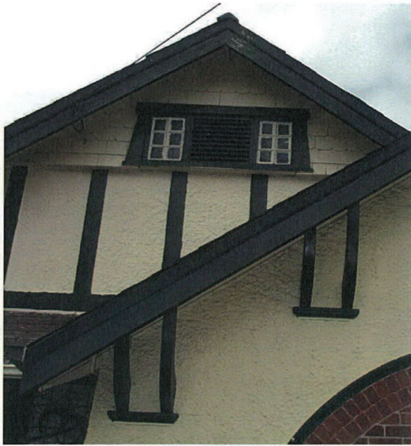
Photo 6: Front gable with attic windows. Stucco Render, Half Timbered detailing, shingled infill & prominent shaped brackets.
