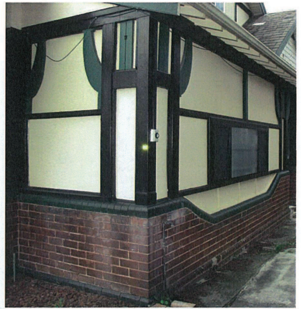
Photo 7: Infill of south side verandah with timber framing and fibre cement. (Reversible)
