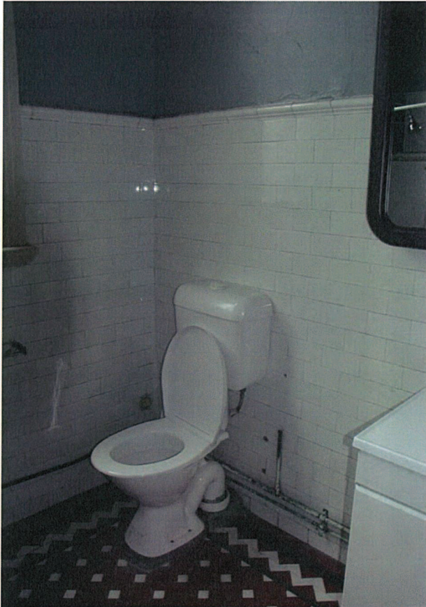
PHOTO 17:EXISTING BATHROOM Retaining original wall and ceiling tiles
