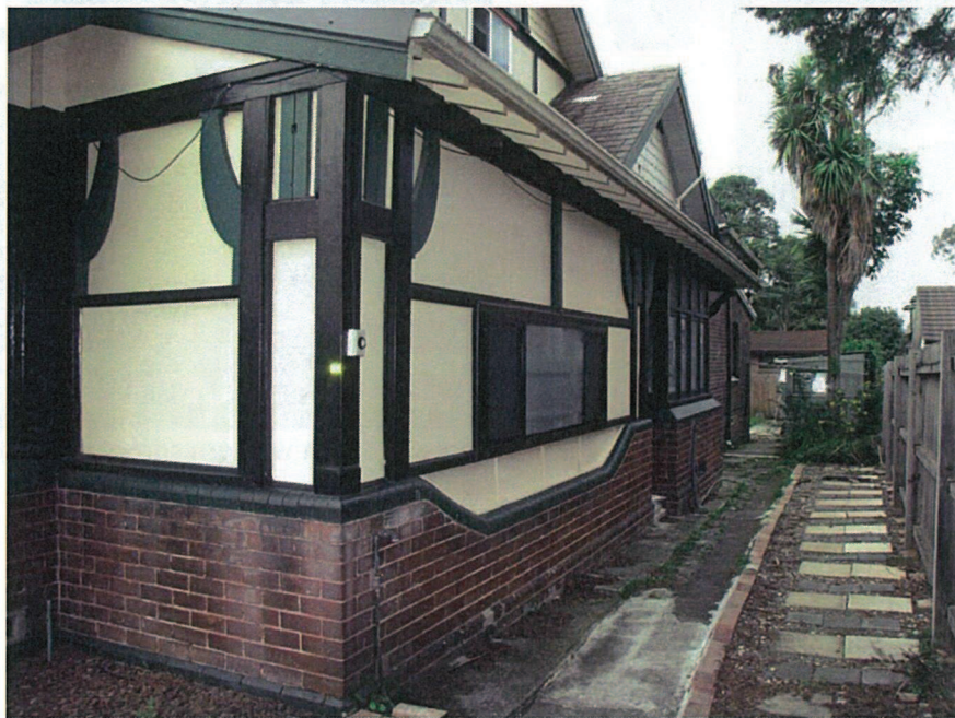
Photo 2: Infill of south side verandah with timber framing and fibre cement. (Reversible)
