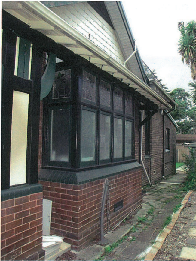
Photo 3: Bay window feature to southern elevation – highly intact.
