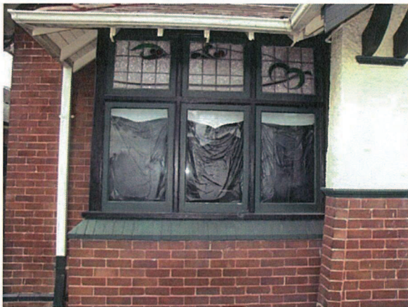
Photo 4: Intact window suite with stained glass toplights.
