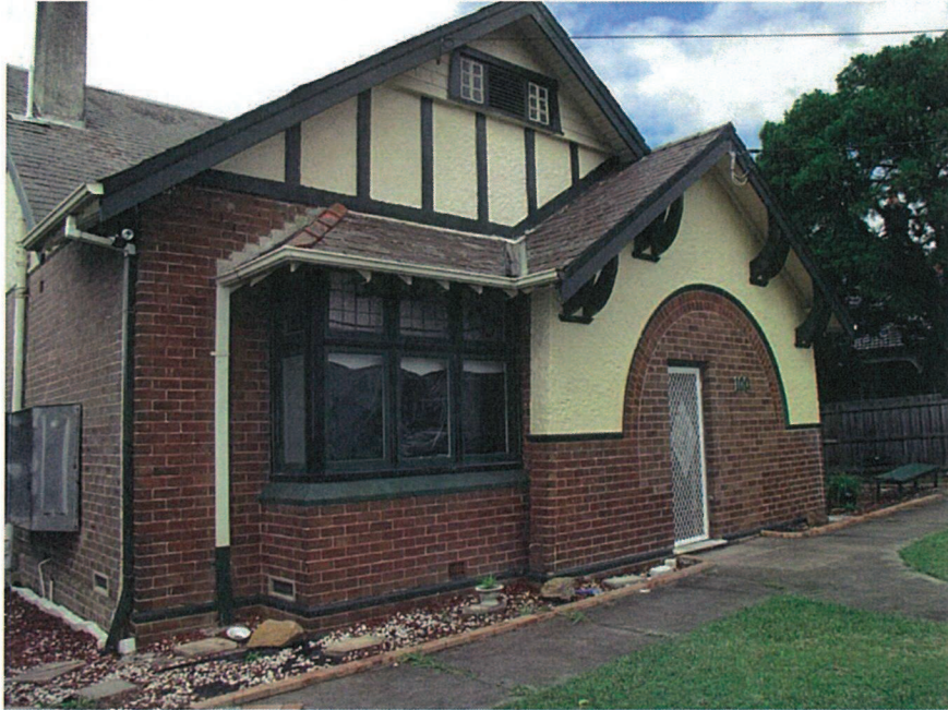
Photo 1: Front (western) Elevation with enclosure to arch of front porch. Roughcast stucco, raking buttress and bracketed eaves indicative of Arts & Crafts influence
